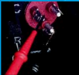
Ohm Out a Compressor
